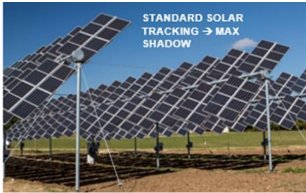
Figure 4: Management of the shadow below Agrovoltaico® tracker 3D
