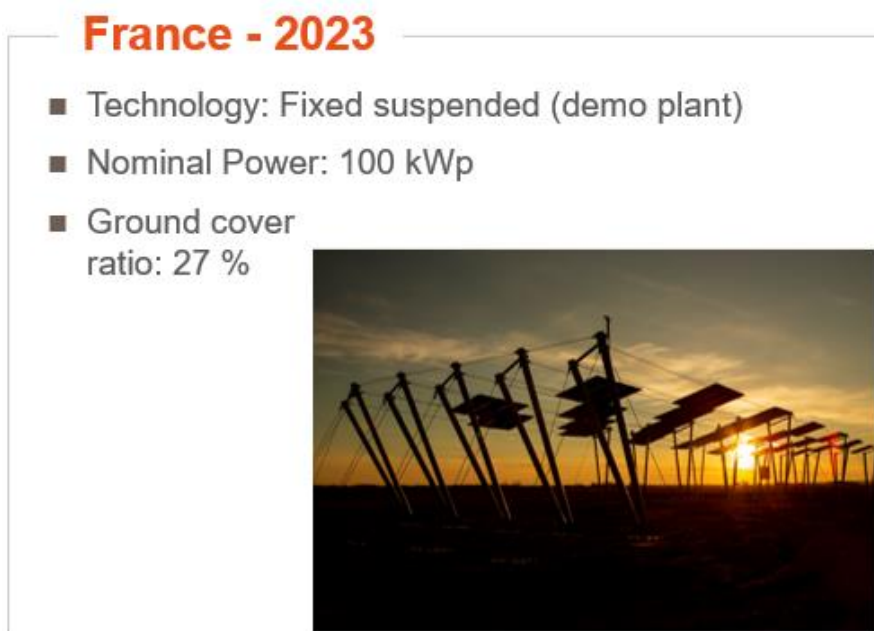
Figure 10: Agrovoltaico® plant in Beaucaire (France)
